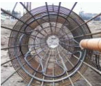
Reinforcement cage with absorber piping and protection tube
